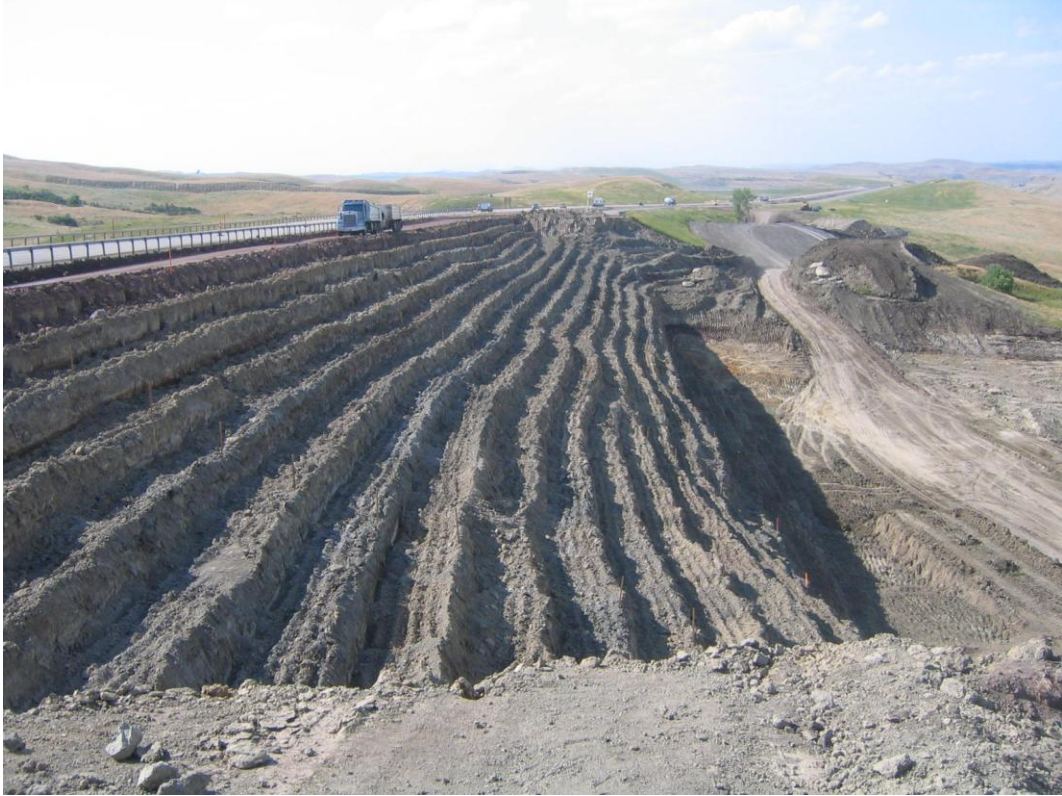
Slide Repair on I-90
