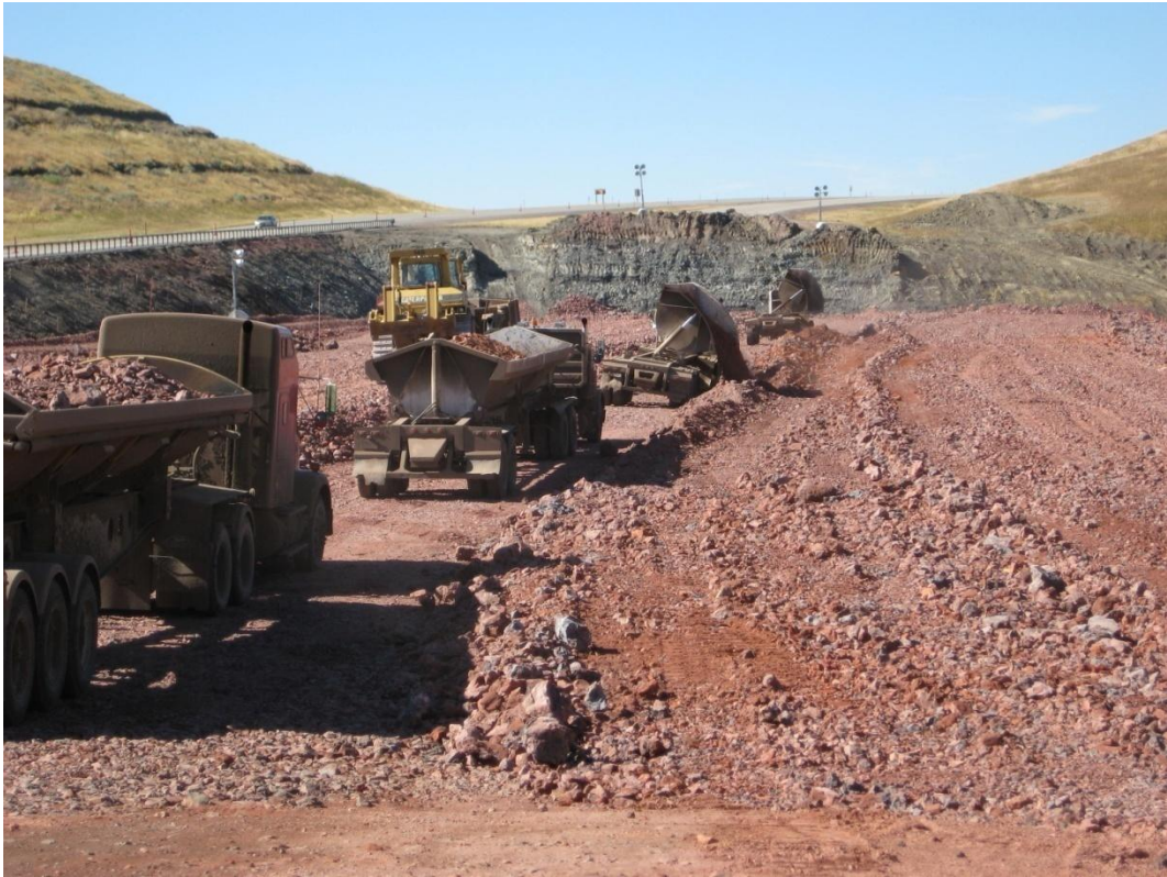
Slide Repair on I-90
